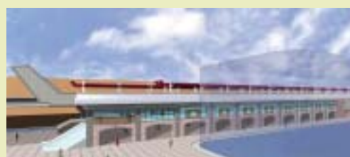
汐止車站 The Sijhi Elevated Station
